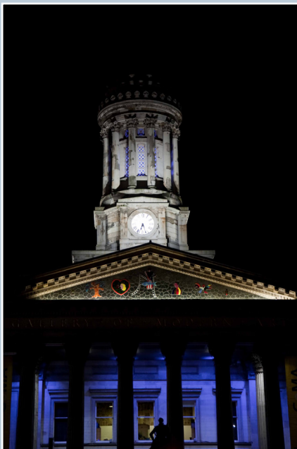
Gallery of Modern Art, Glasgow. The floodlights are positioned behind a cornice and on the roof, therefore making little impact in daylight but providing atmospheric lighting after dark. © N. Haynes.
