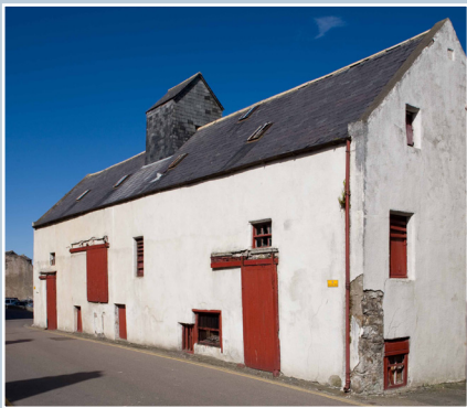
Sliding boarded doors on a late 18th-century granary building in Banff, Aberdeenshire. © N. Haynes.
