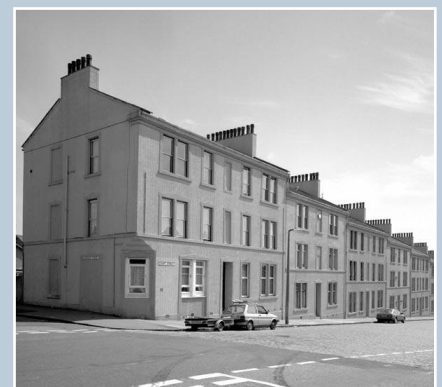
Mass concrete tenements in Dundee, cast insitu in 1874–5 by the Concrete Building Company for the Working Men's House Building Association. The buildings were renovated and a buff render applied in 1982–4. © Crown copyright: RCAHMS. Licensor www.rcahms.gov.uk .
