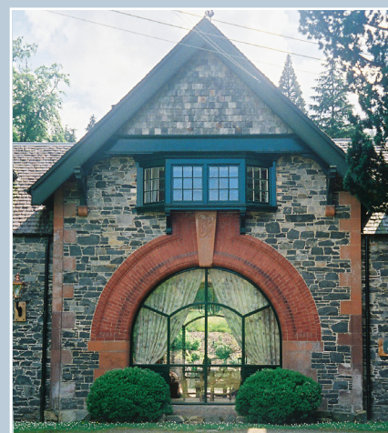
Dawyck Stables, Bellspool, Scottish Borders, after conversion. The original door opening has been retained, but glazed to allow for residential use.
