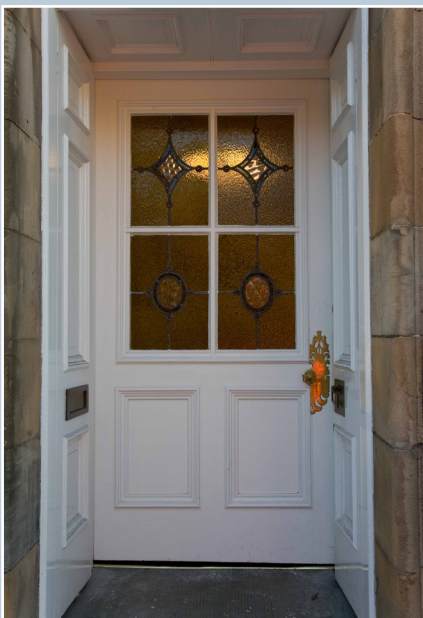
A late 19th-century two-leaf outer door and an inner vestibule door with decorative leaded glass panels in Falkirk. Associated fixtures include the brass letterbox and door handle on the outer door and the brass doorknob and decorative finger-plate on the inner door. © N. Haynes.
