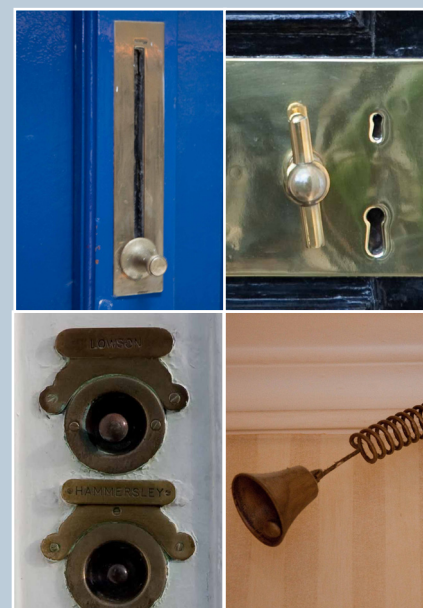
Associated fixtures (clockwise from top left): tenement door release (1890s); brass handle and lock (1880s); door-bell (1890s); door-bell pulls (1820s). © N Haynes.
