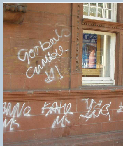
Graffiti: The removal of graffiti requires prompt action before the paint or ink dries into the wall surface. Cleaning methods should be tested on a small unobtrusive area to determine the least aggressive treatment for effective removal of the graffiti. In extreme cases of repeated vandalism, a sacrificial wax coating might be considered for vulnerable surfaces.
