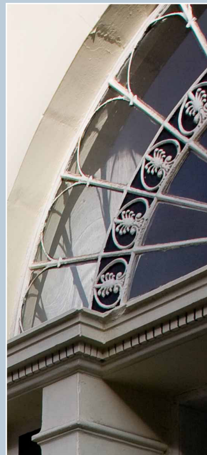
Detail of a delicate cast-iron fanlight dating from the 1790s in Edinburgh. © N. Haynes.
